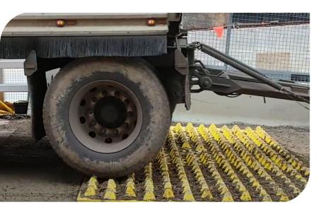
The site crew converted to FODS mats after seeing its results with traction despite being on an incline, even when conditions were wet and muddy.
