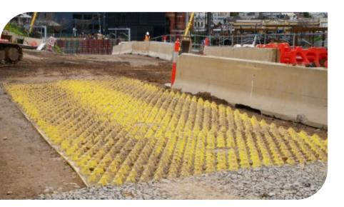
The nature of the mats allowed the team to construct the stretch of mats away from the access road and then drag the FODS into place once it was assembled. This meant the project did not stop the flow of traffic to install.
