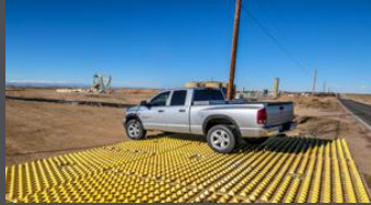
Resources & Energy Sectors
